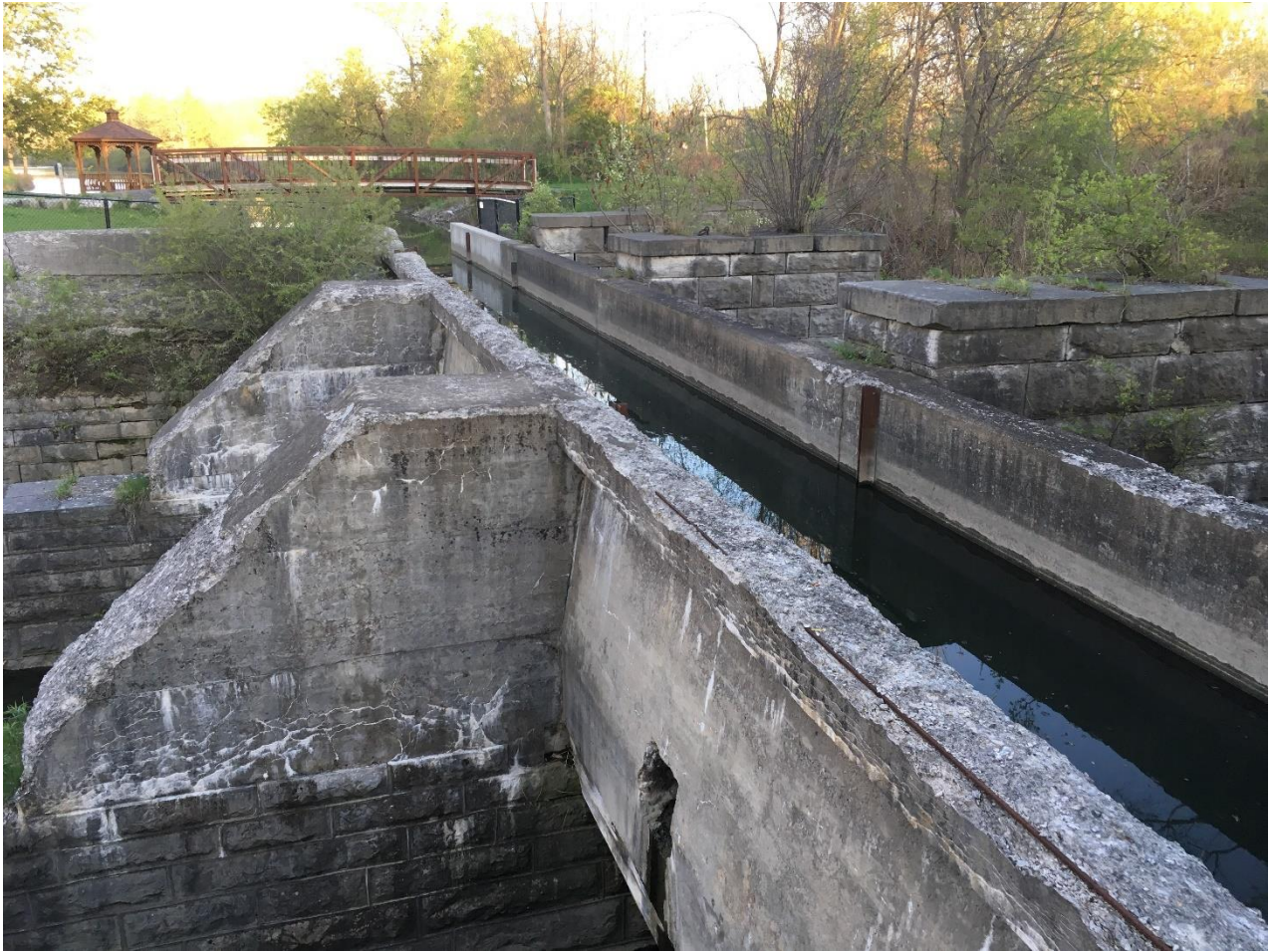
Photograph of the Butternut Creek Aqueduct.
